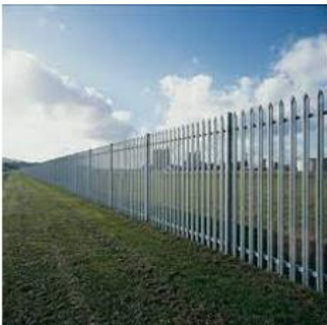
Plate 4-12. Standard palisade fencing
