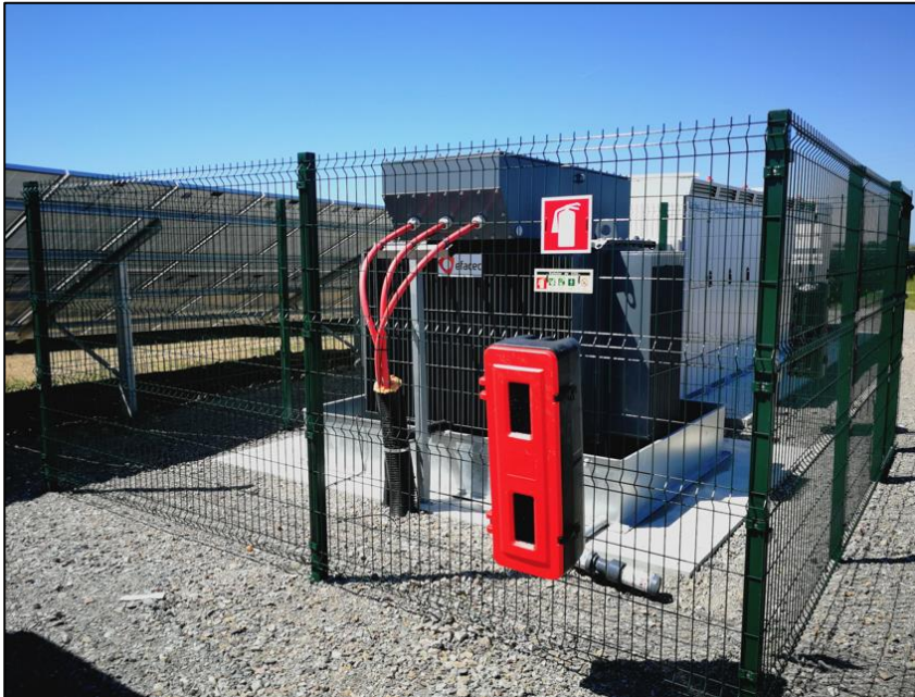
Plate 4-11. Typical transformer compound fencing
